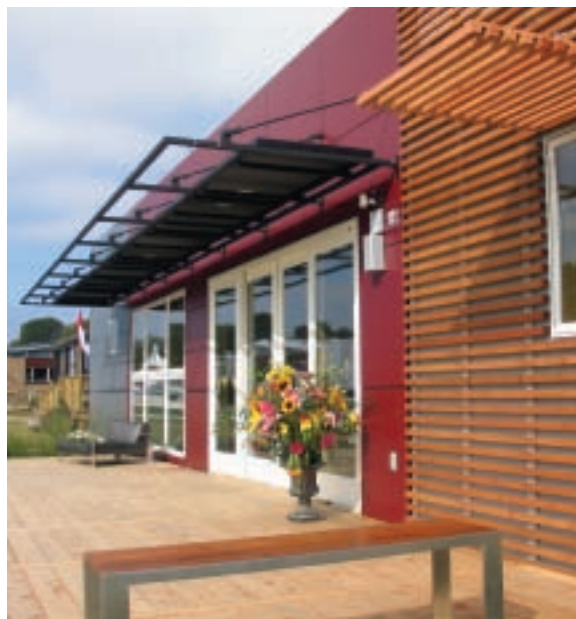
[Below] The PV module awning shades the tank from the higher summer sun. The Trombe Wall then acts as a source of “coolth,” and absorbs heat from the house. The PV modules can be moved back and forth to shade the window or let the sun shine on it.
