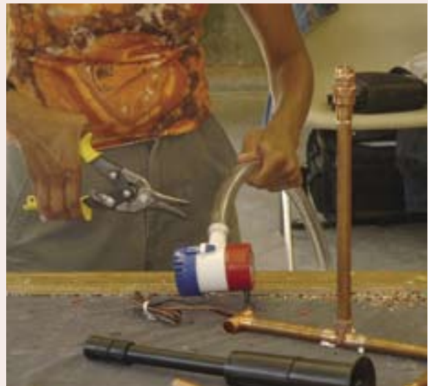
A pump is attached to the copper pipe and wired to a solar-electric module.
