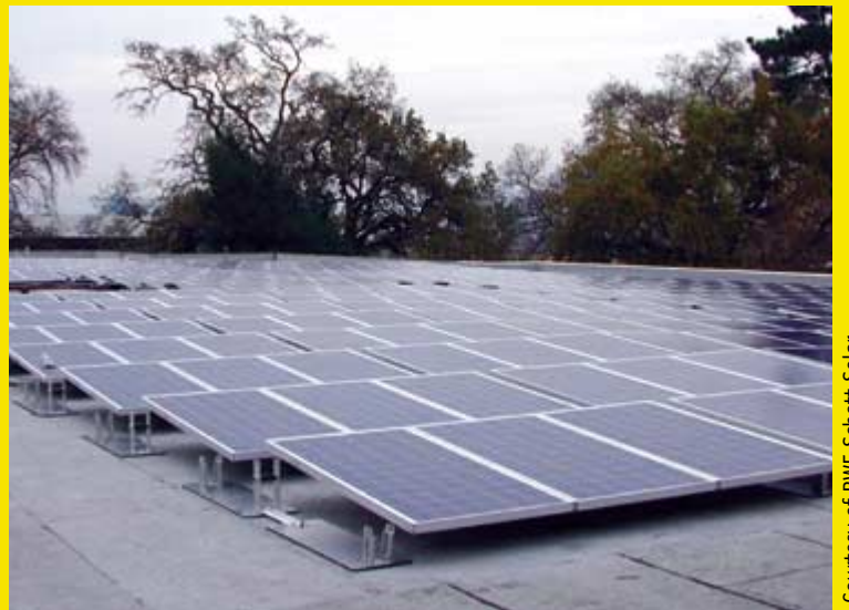
A free-standing solar panel roofing material that just sits on the roof without any adhesion, without drilling supports into the roof, and yet can withstand winds of over 110 miles per hour.
