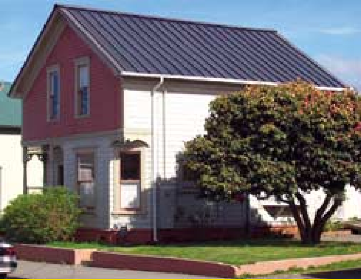
For this Eureka, California building, flexible panels are attached to a standard roof deck.
