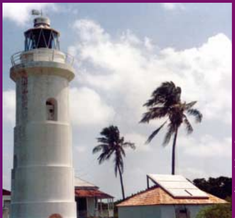
Courtesy of Automatic Power, Inc.
