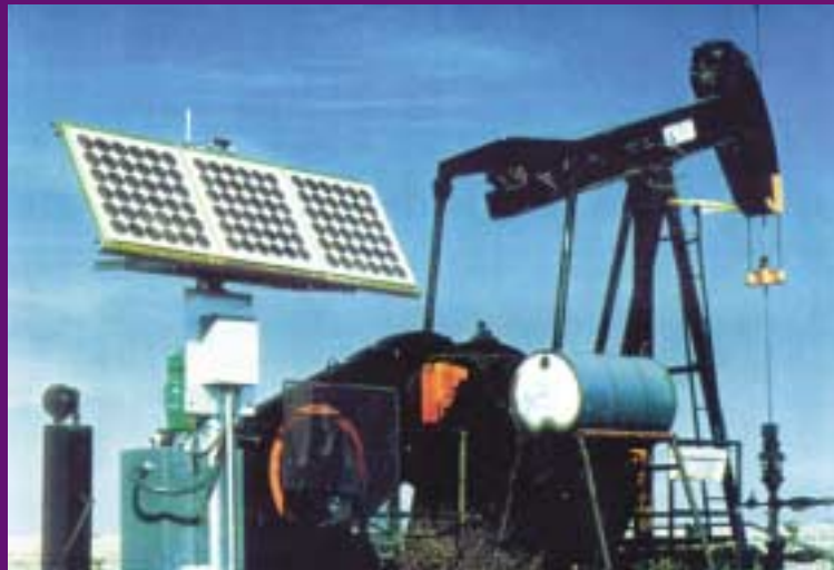
Courtesy of Solar Power Corporation
