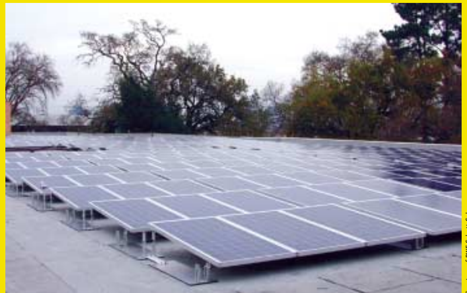
A free-standing solar panel roofing material that just sits on the roof without any adhesion, without drilling supports into the roof, and yet can withstand winds of over 110 miles per hour.
