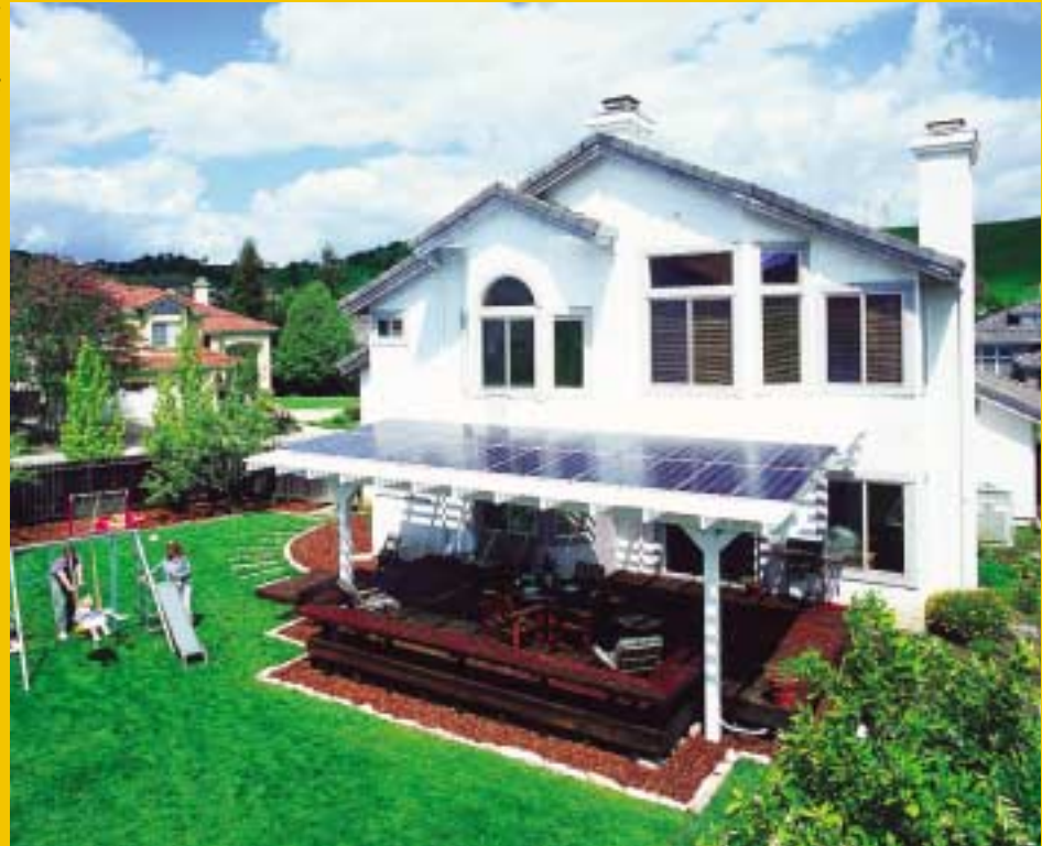
One of many homes in California now with solar electricity. This solar array, installed on a patio trellis, provides shade while producing energy to power the home.
